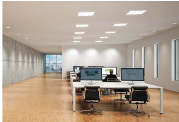
10:30 Artificial lighting is turned down as more daylight becomes available and the light colour is made more intermediate
